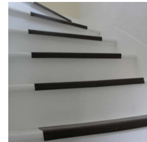
After lead paint interim controls
