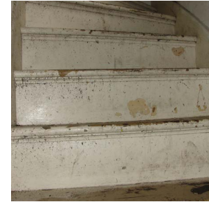
Before lead paint interim controls
